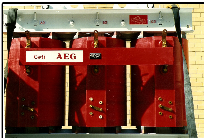
22kV 0.5MVA Cast Resin Transformers
